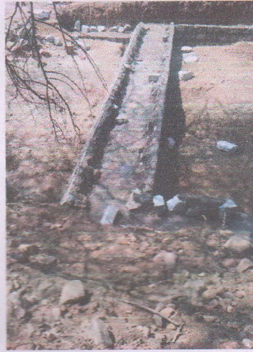
During work - Earth work and RR Masonry Work
