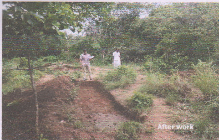
DFO INSPECTION AND CHECKING MEASUREMENTS
